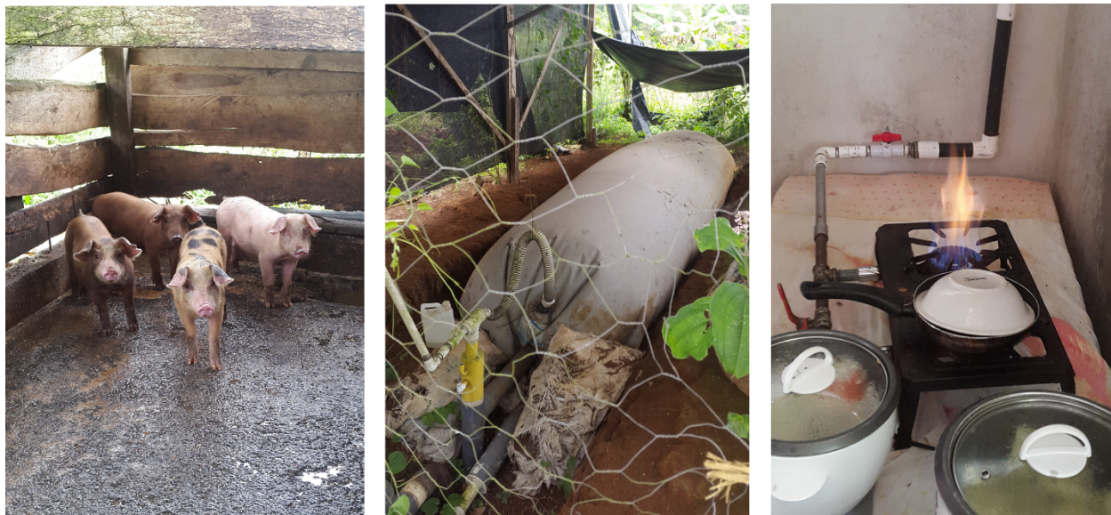
Figure 1 Left) Pig stall with pigs, Middle) filled pressurized biodigester bag and Right) burned methane flame.
